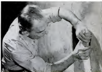
Remove old finish before damp-proofing.
